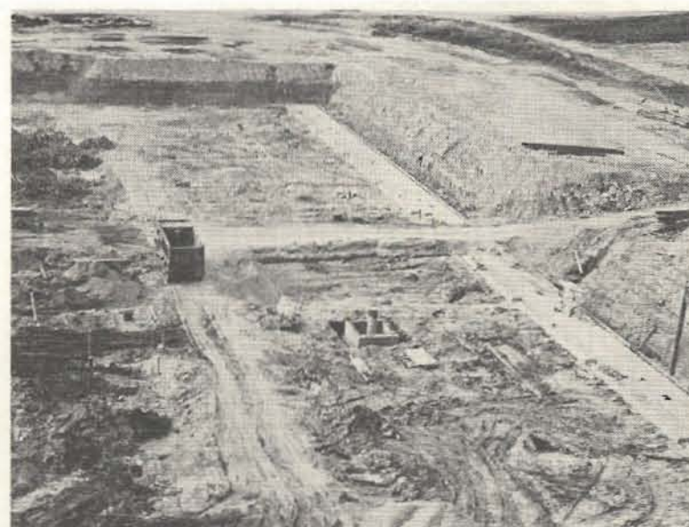
WORK PROGRESSES ON HEALTH EDUCATION BUILDING
