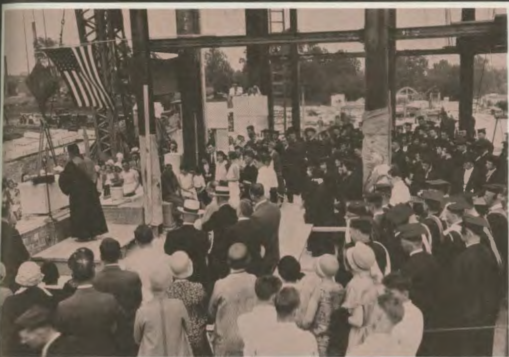
University Hall Cornerstone Laying, June 12, 1930 President Doermann speaking beneath the flag
